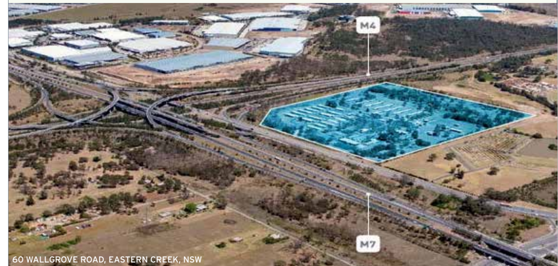
60 WALLGROVE ROAD, EASTERN CREEK, NSW
