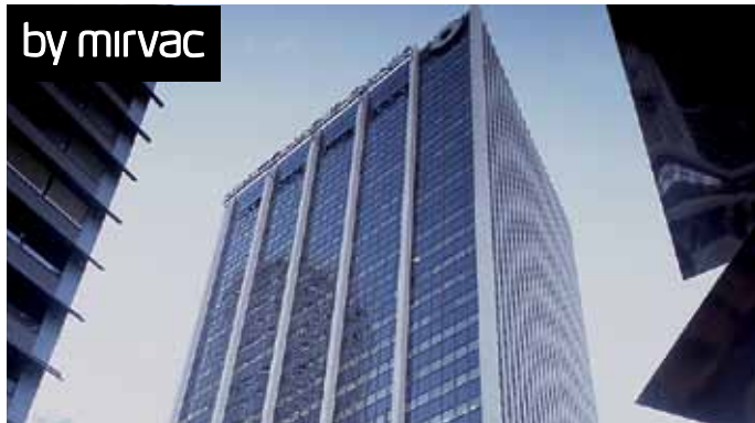
10 - 20 BOND STREET, SYDNEY, NSW IN PROGRESS
