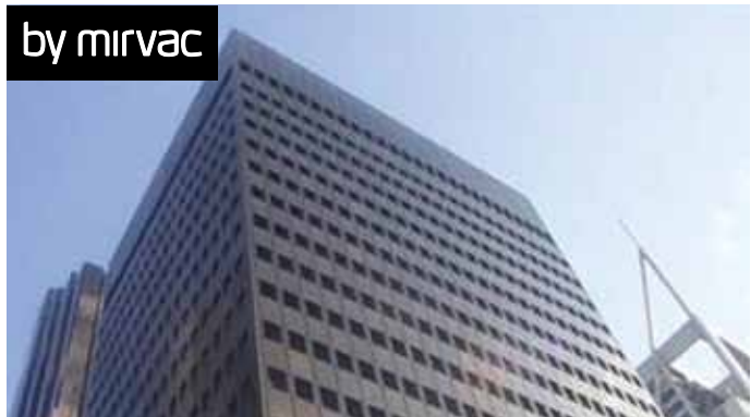
8 CHIFLEY SQUARE, SYDNEY, NSW IN PROGRESS
