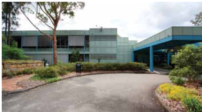
55 COONARA AVENUE, WEST PENNANT HILLS, NSW
