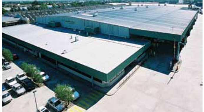
44 BILOELA STREET, VILLAWOOD, NSW 1
