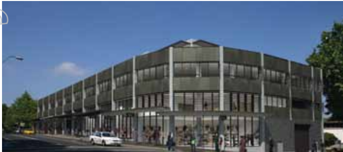
SYDNEY WATER, SURRY HILLS, NSW COMPLETED
