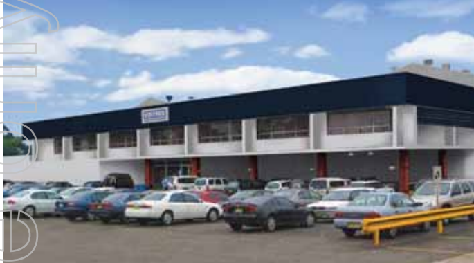
64 BILOELA STREET, VILLAWOOD, NSW
