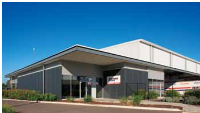
32 SARGENTS ROAD, MINCHINBURY, NSW
