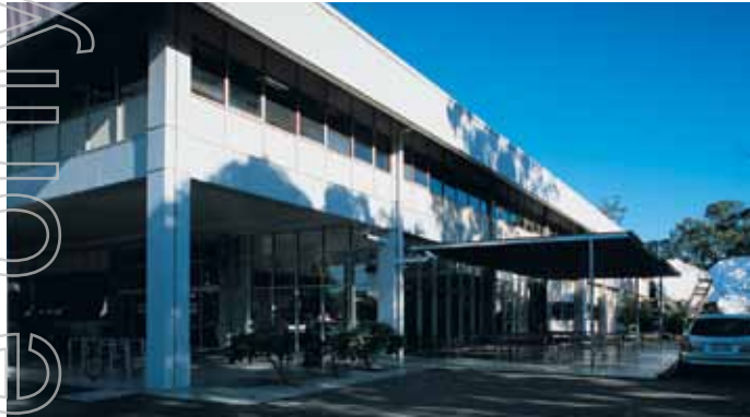
271 LANE COVE ROAD, NORTH RYDE, NSW
