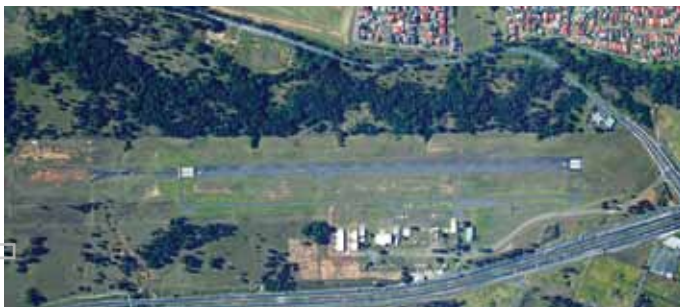
HOXTON PARK AIRPORT, INTERSECTION OF M7 AND COWPASTURE ROAD, HOXTON PARK, NSW 1 PROPOSED
