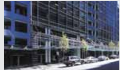
40 Miller Street, North Sydney, NSW $93.5m 12,664 sqm NABERS Energy rating: 4 Star
