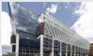
Sirius Building, 23 Furzer Street, Canberra, ACT $225m 46,167 sqm 5 Star Green Star Office Design
